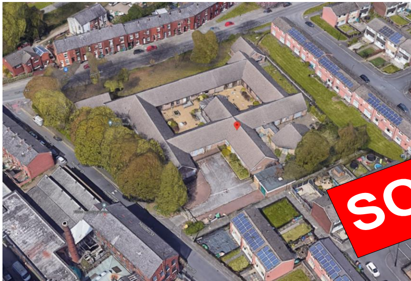
Kingsfield Care Home, Union Road, Ashton under Lyne
